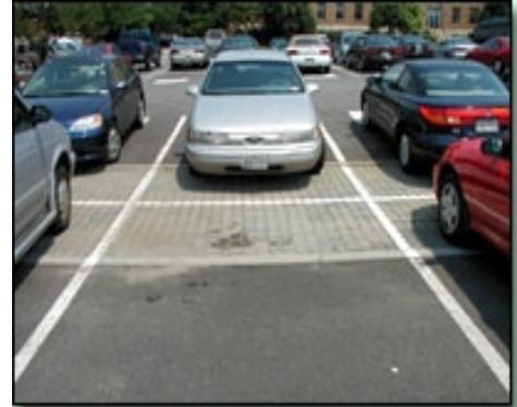
Porous pavement can help to reduce the increased temperature commonly associated with increased impervious cover.
