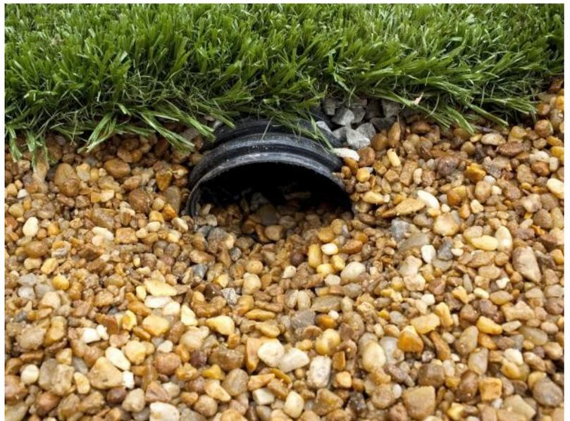
*French drain daylighting onto a pile of gravel. Source: HGTV.*
