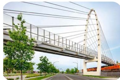
University Gateway Bridge Pullman, WA Length- 450'
