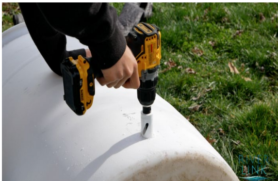
Figure 21 Drilling a hole for the spigot
