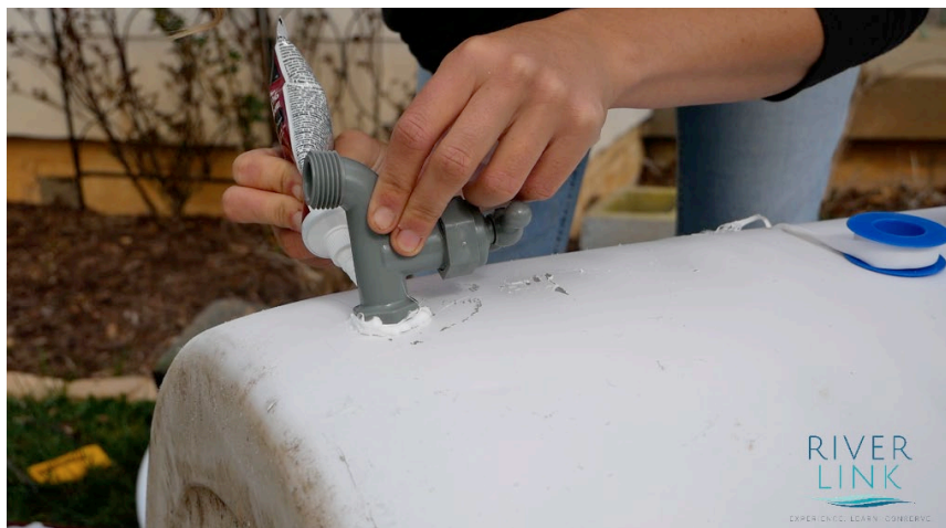
Figure 23 Caulking spigot
