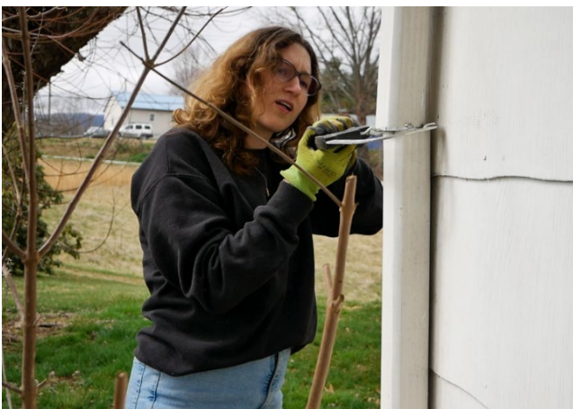
Figure 24 Cutting the gutter downspout
