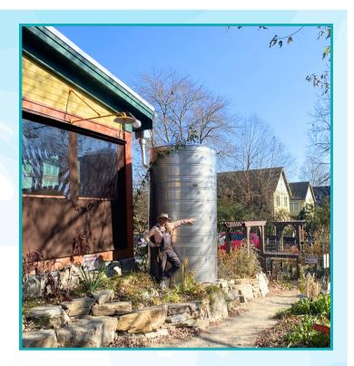
Until recently, Asheville's Sunny Point Cafe dealt with flooding issues caused by roof runoff. This flooding impacted their outdoor dining space and parking lots. Then in 2022, their Garden Manager, Alice, worked to redirect the problematic roof runoff into a series of rain barrels. Their rain barrels vary in size from 125 to 2000 gallons. The water collected in the rain barrels is now used to irrigate their garden beds.
